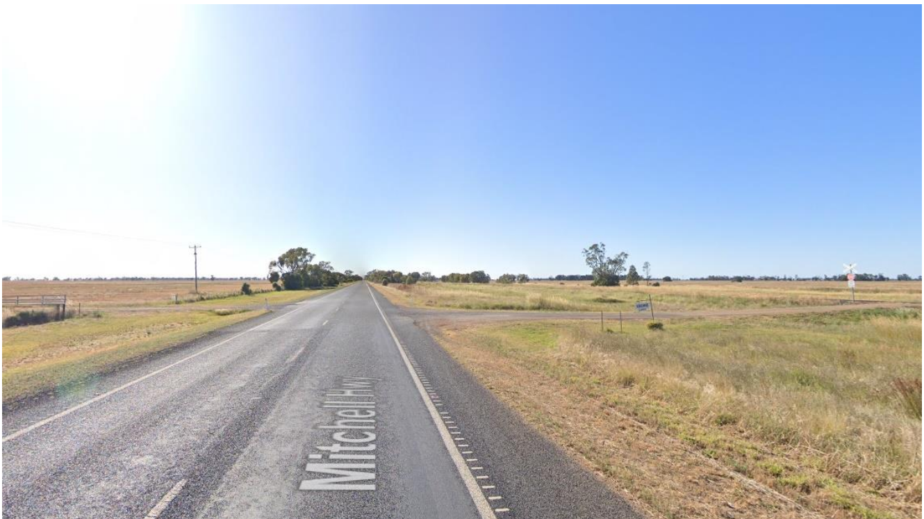
Figure 4: Mitchell Highway facing southeast adjacent to the subject site access on the left (Source: Google)
